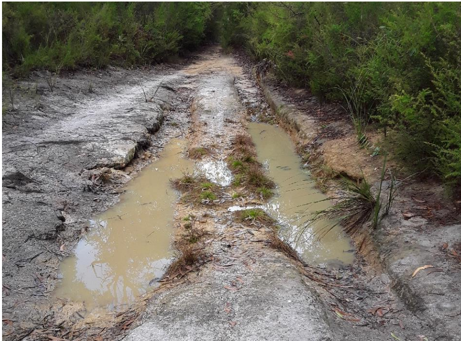
Image 29: Example of erosion along internal tracks (May 2023).
