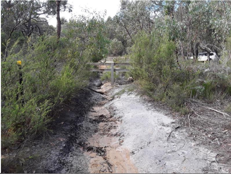
Caption: Erosion at track entrance that needs to be remediated (next to photo monitoring point 2 – left hand side of photo).
