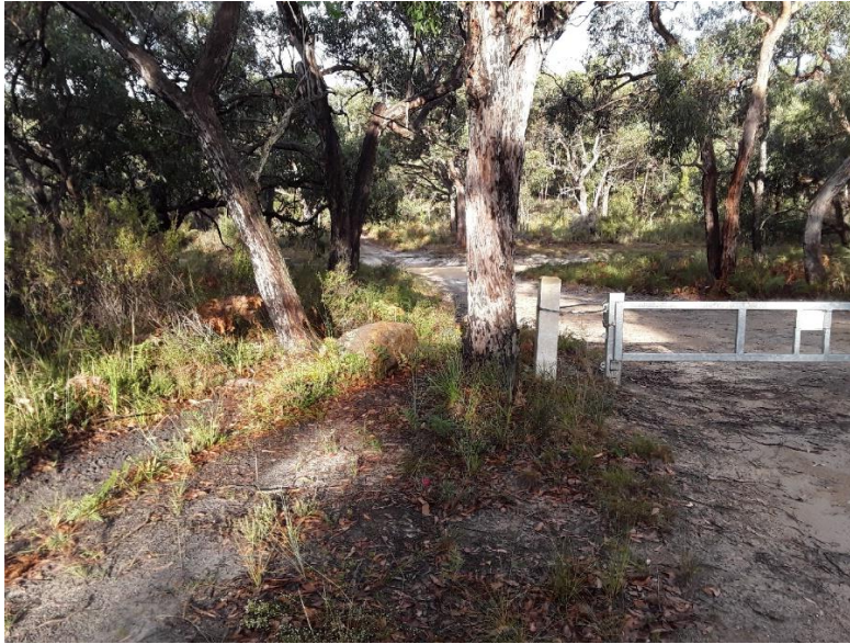
Image 5. Boulders have been installed either side of the northernmost gated track entrances from Distillery Creek Road (left hand side of gate shown here) to prevent illegal access. Trail bike tracks either side of boulder indicate that bikes are bypassing these boulders and the gate (also see Image 6) (May 2023).
